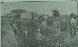
LAYING HENLEY'S CABLES IN DURBAN.
