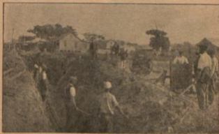
LAYING HENLEY'S CABLES IN DURBAN.
