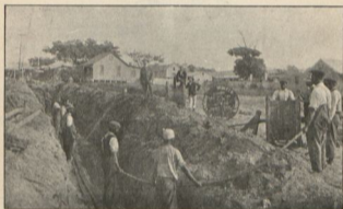
Laying Henley's Cables in Durban.
