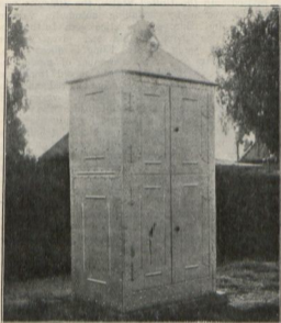
PRESSED STEEL TRANSFORMER KIOSK: CAPACITY 100 K.V.A.
