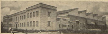
The South African General Electric Factory at Benoni, Transvaal
