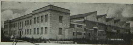
The South African General Electric Factory at Benoni, Transvaal
