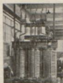
No. 434-1. The assembly of a 600 kVA Farnace Transformer. H.V. 8,600 volts, L.V. 55 volts 3,600 amps. Transformer fitted with off-load tap changer. Weight of unit 5 tons.
