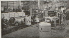
Welding electrodes leave the oven after baking, ready for inspection and packing.
