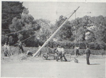
Fig. 2 CONCRETE POLE ERECTION.
