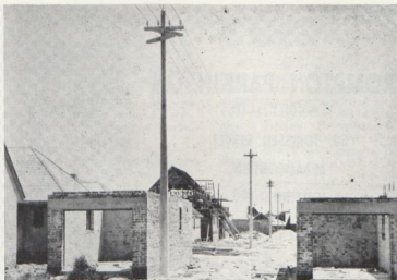
MID BOUNDARY CONSTRUCTION DURING BUILDING OPERATIONS
