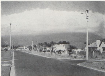
MID BOUNDARY CONSTRUCTION—STREET SCENE.
