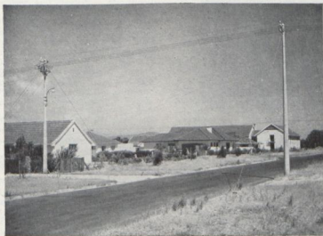
MID BOUNDARY CONSTRUCTION—ROAD CROSSING.
