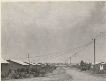
PHOTOGRAPH A. Overhead House Service Connections
