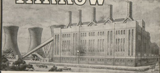
13th Avenue Power Station, Bulawayo, Southern Rhodesia.
