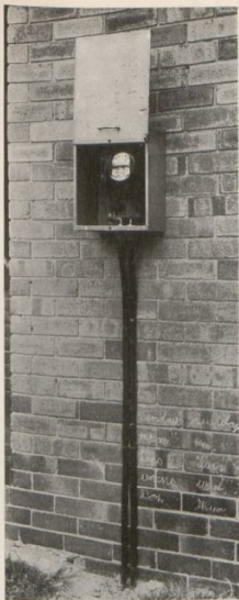
PHOTOGRAPH E. Typical Underground Service Connection at Orlando East.
