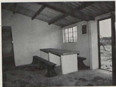
No. 9. Bachelor Hostels. View in kitchen showing position of distribution board and 4-gang switch in passage.
