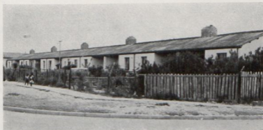
No. 2. Later type of Married Quarters with 3-phase supply to blocks and common metering point.
