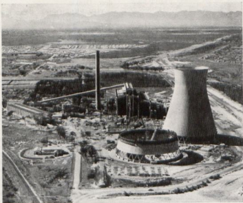
A view of Athlone Power Station under construction for Cape Town City Council
