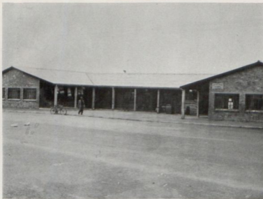
No. 11. New shops, 1958, showing centre block.
