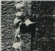
FIGURE 4: Particle inclusion between screen and insulation in polyethylene cable
