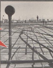
A DECKING WITH PVC CONDUIT, PRIOR TO CONCRETE BEING THROWN
