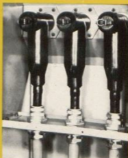
Stress cones terminating 3 core cable
