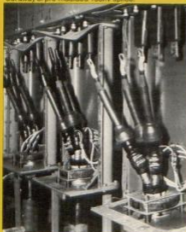
Switchgear terminations
