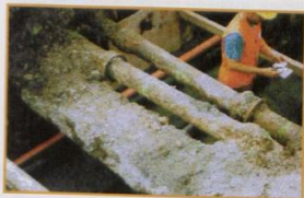
Figure 6. Services Crossing the Cable.
