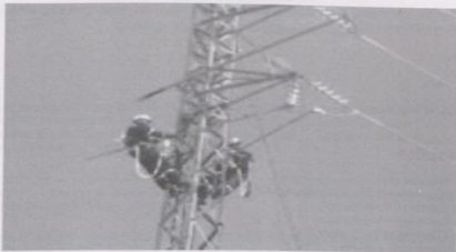
Figure 3. Stick Method working from the structure
