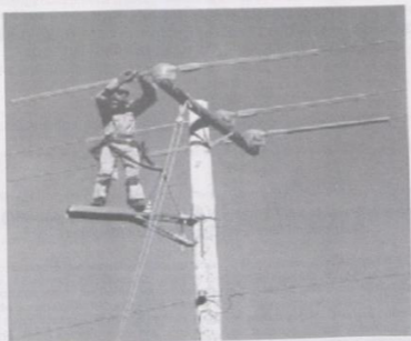
Figure 1. Gloving Method working from an Insulating Platform
