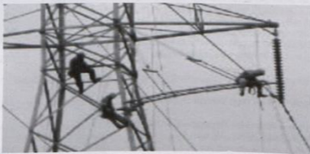
Figure 4. Barehand Method working from the insulating ladder
