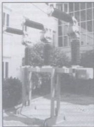
Integrated SF6 Unit CB 90° to CT (Fig 4)
