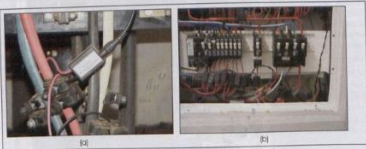
Fig. 8: Different coupling methods: (a) Capacitive and (b) inductive.
