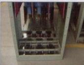
Fig. 10: Provision for each incoming cable on 2500 A panels.
