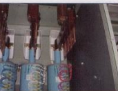
Fig. 10: Provision for each incoming cable on 2500 A panels.
