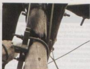
Fig. 4: The initial tracking on wood surface in areas where pollution plays a role can be seen in Fig. 4(a). The ignition of the wood and destruction of the structure can be seen in Fig. 4(b). The leakage current is a function of the pollution in the area, the type of insulators used on the structure and the number of parallel leakage paths that are available on the structure.
