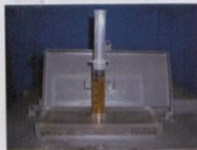
Fig. 5: Test access cover plate and sample kit fitted on a ring main unit.
