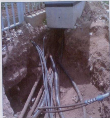
Fig. 1: The joint pit.
