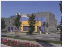
Fig. 4: Geothermal plant in Bavaria (40 MW heat, 3,4 MWe)
