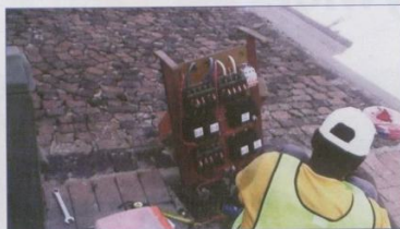
Fig. 4: ULM Remote master installation in Kiosk or stubby box.
