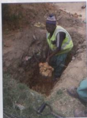
Fig. 2: The planting of an electric pole by a local labourer.
