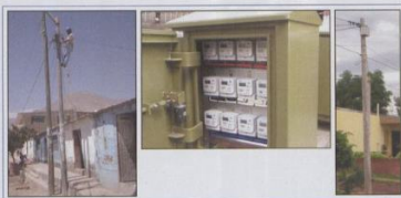
Fig. 2: Variety of types and locations of enclosures for split prepayment meters.
