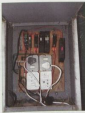
Fig. 2: Pictures of unsafe conditions of electricity circuitry within the caravan park.
