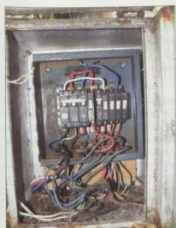
Fig. 2: Pictures of unsafe conditions of electricity circuitry within the caravan park.
