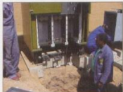
Fig. 18: Example of SF6 RMU with an additional raising plinth and removable front sections.
