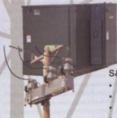
IntelliSwitcher® Pulse-Closer Pad-Mounted and Pole Mounted Installation Styles
