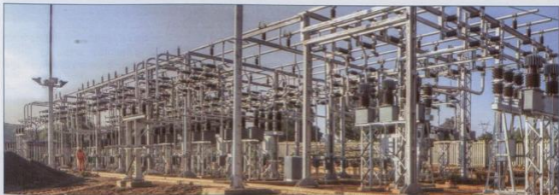
Fig. 1: Condale substation upgrade.
