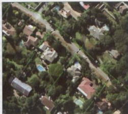
Fig. 3: Aerial view of assets.
