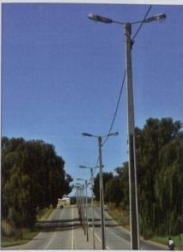
The Brooklyn/Springs road where vandai-prone steel street-lighting poles have been replaced with prestressed concrete poles.
