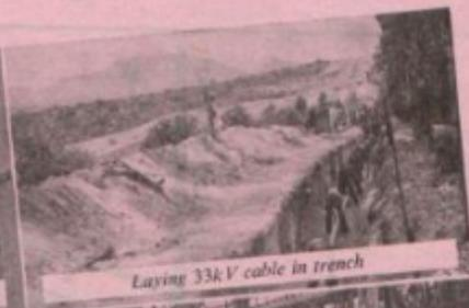
Laying 33kV cable in trench
