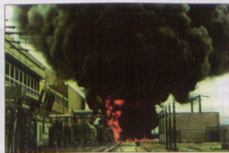
Fig. 1: Transformer fault due to a defective bushing.
