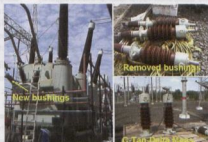
Fig. 21: 33 kV OIP bushings.
