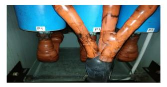
Fig. 7: Cable termination @ 11 kV switchgear panel
