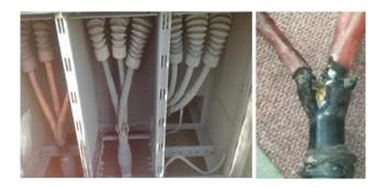
Fig. 12: 11 kV switchgear cable termination failure
