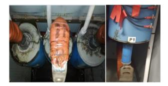
Fig. 8: Tracking CT's @ 11 kV switchgear panel
