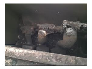
Fig. 13: 11 kV Busbar failure
