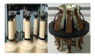
Fig. 6: Cluster contact @ 11 kV switchgear panel
