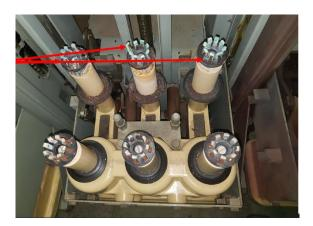
Fig. 9: Cluster contact @ 11 kV switchgear panel
