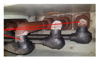
Fig. 10: busbar - bushing connection @ 11 kV switchgear panel
