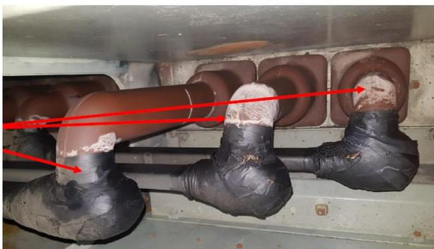
Fig. 10: busbar - bushing connection @ 11 kV switchgear panel
