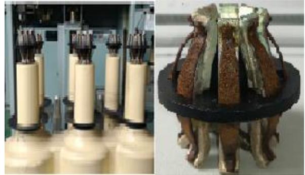
Fig. 6: Cluster contact @ 11 kV switchgear panel
