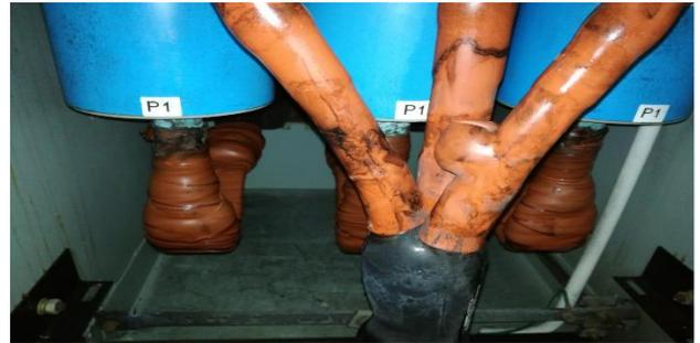
Fig. 7: Cable termination @ 11 kV switchgear panel
