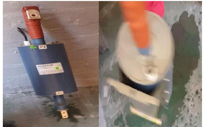
Fig. 11: Tracking CT's @ 11 kV switchgear panel
