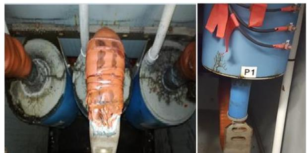
Fig. 8: Tracking CT's @ 11 kV switchgear panel
